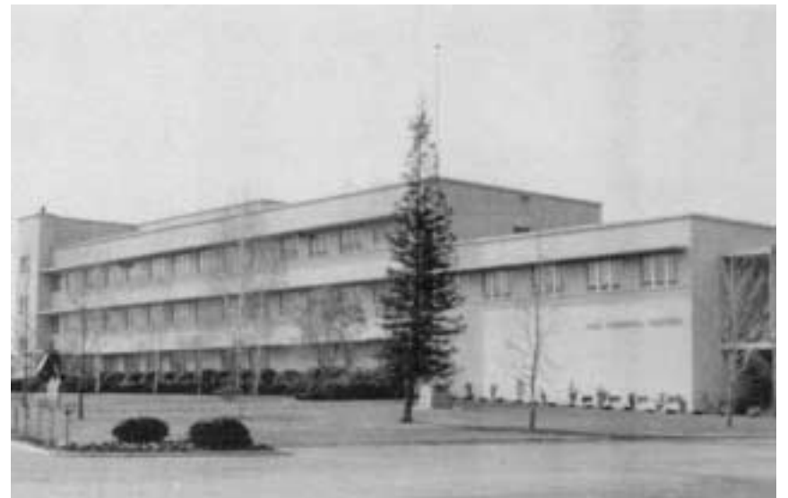
View of the hospital in 1964.
